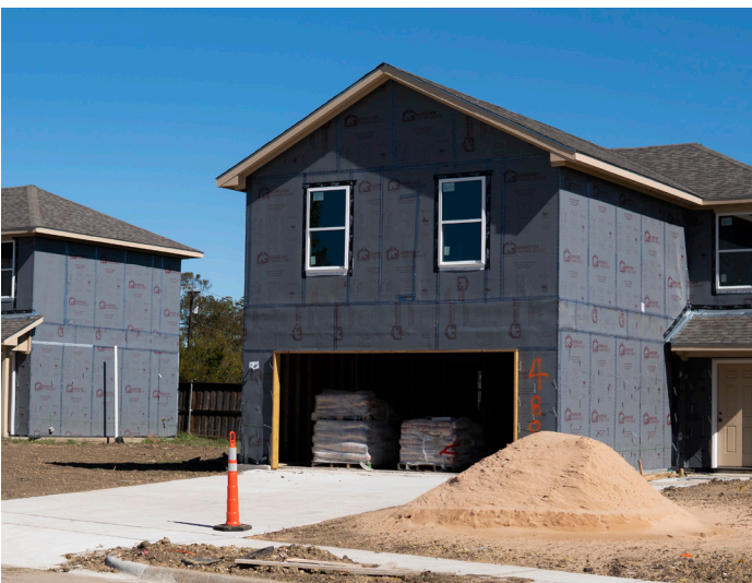
New housing development in Sherman
