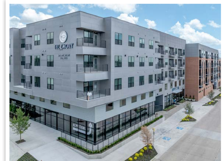
The Emory apartments recently completed at the former Plano First Baptist Church site, which is being redeveloped (Map #36j)
