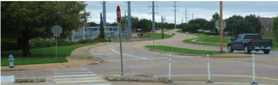
Wilson Creek Parkway from Towne Lake
