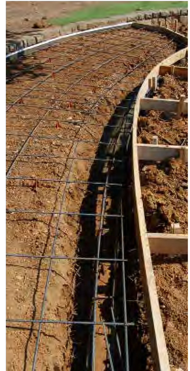
Trail Under Construction
