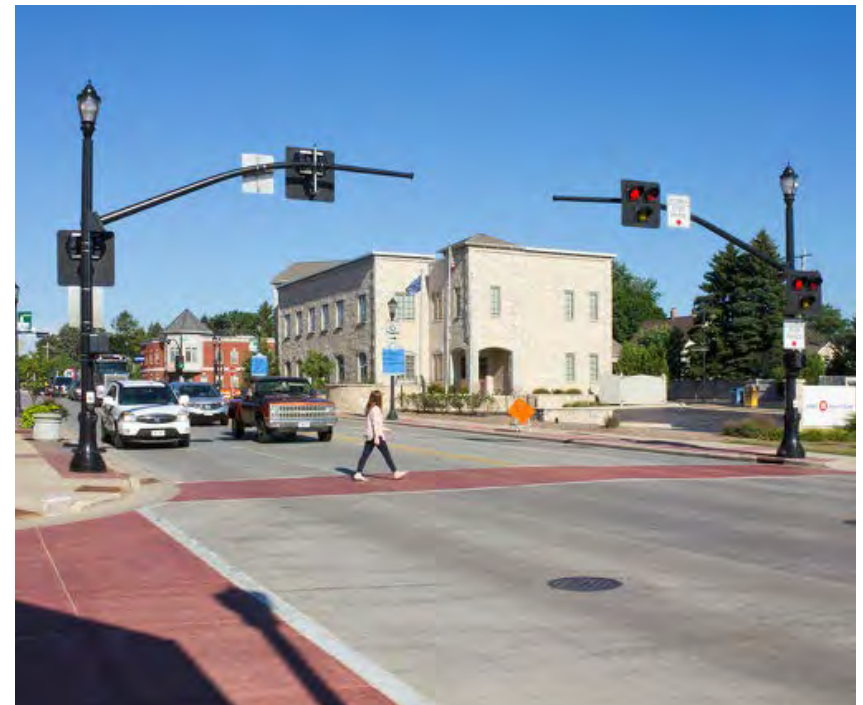
Signalized Crossing - HAWK Signal
