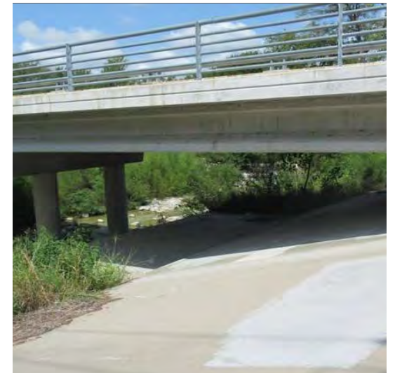
Terraced Abutment at Silverado
