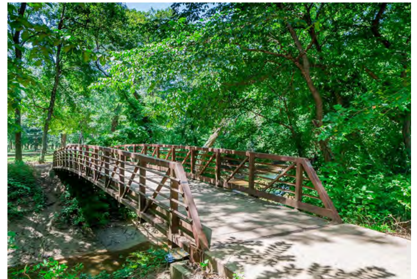
Sidewalk Segment on McDonald Road
