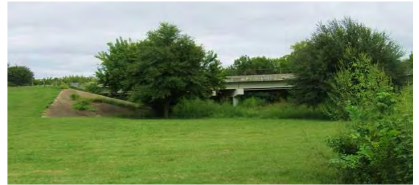
Eldorado Bridge at Wilson Creek
